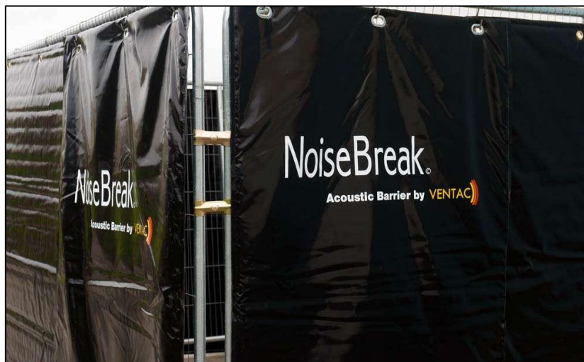
Figure 13: Temporary Construction Noise Barrier © Ventac
