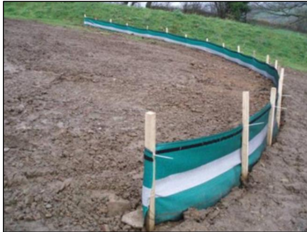
Figure 11: Typical Silt Fencing
