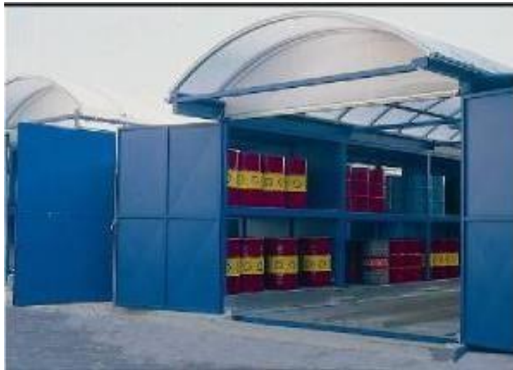
Figure 16: Safe Storage, Bunded and Under Cover
